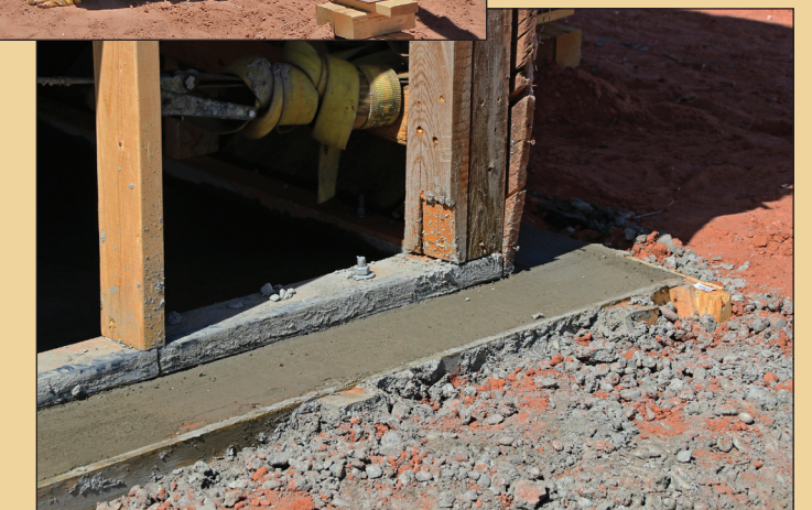
New concrete hardens at a corner of the trading post.
