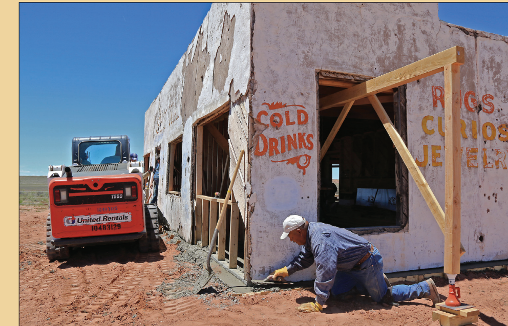
As concrete filled the trench, workers troweled it to a smooth finish.
