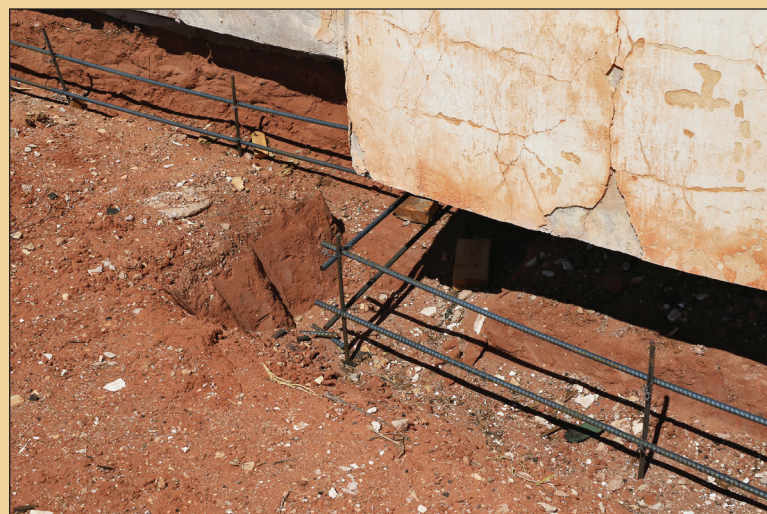
Bottoms of exterior walls were trimmed to match the level of the slab floor inside.
