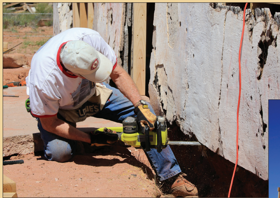
Bottoms of exterior walls were trimmed to match the level of the slab floor inside.
