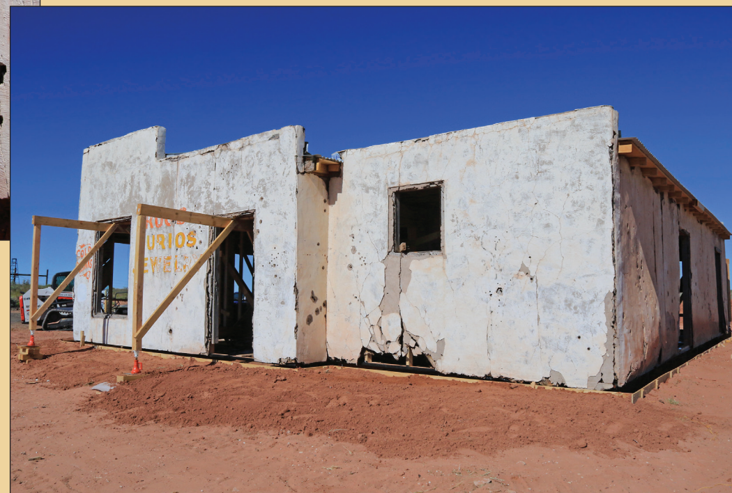
Once set, the concrete forms were backfilled with earth for support.
