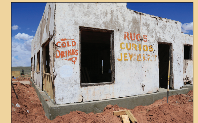
Forms were removed the following day, revealing the new foundation.
