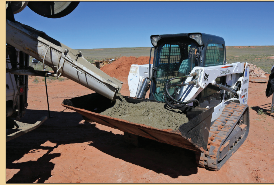
Specialized equipment was used to maneuver the wet concrete.
